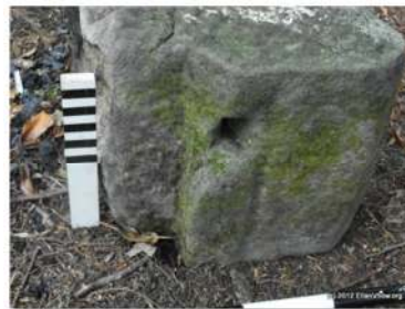
Figure 3 – A finished stone, part of a castle window, was discovered this summer. A vertical groove, designed to receive leaded glass, is clearly visible. Note also the socket for an iron bar to support the leaded glass.
