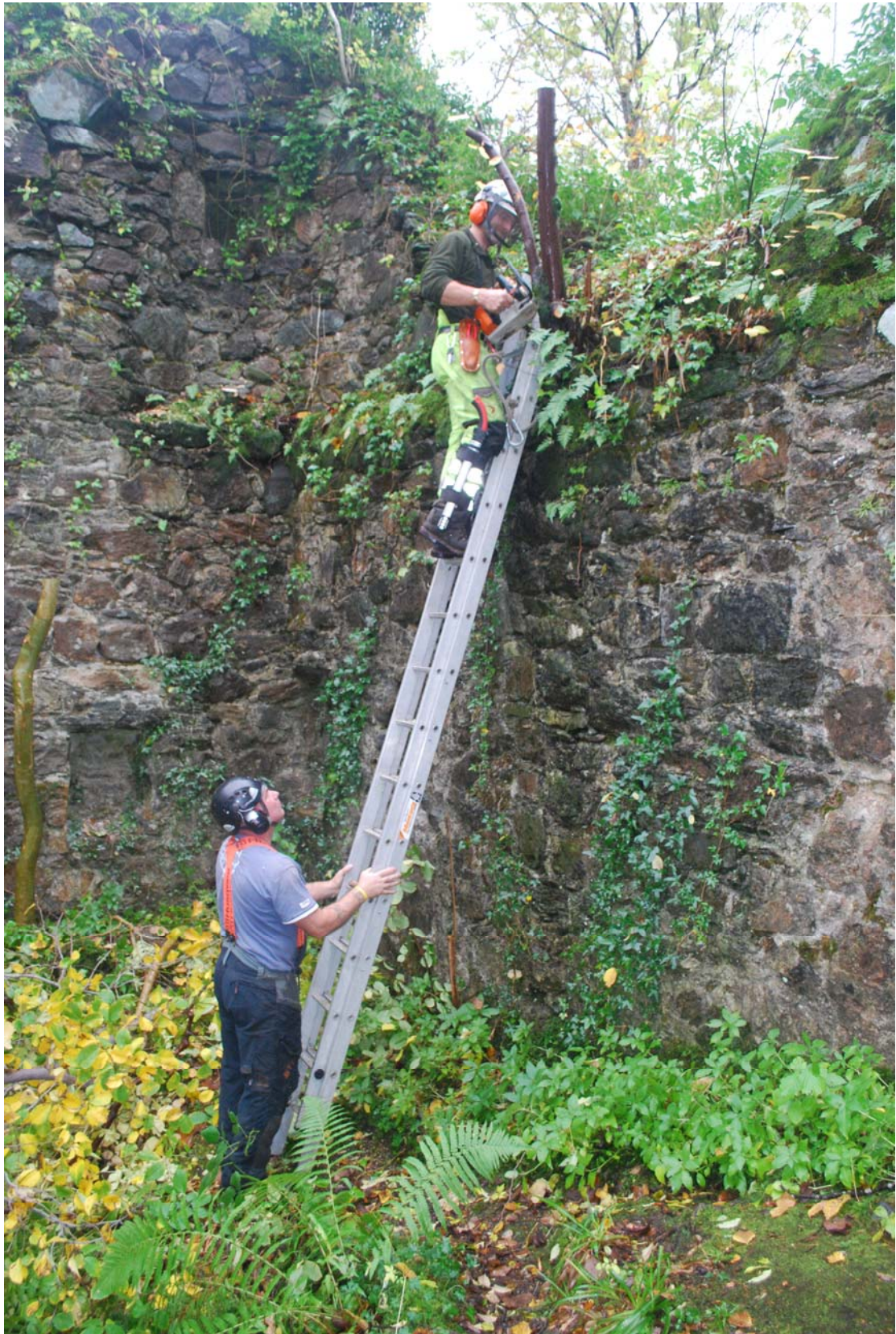
View to ESE, Felling saplings on the S wallhead (Liam Mackenzie up ladder and Derek Triplett holding ladder).
