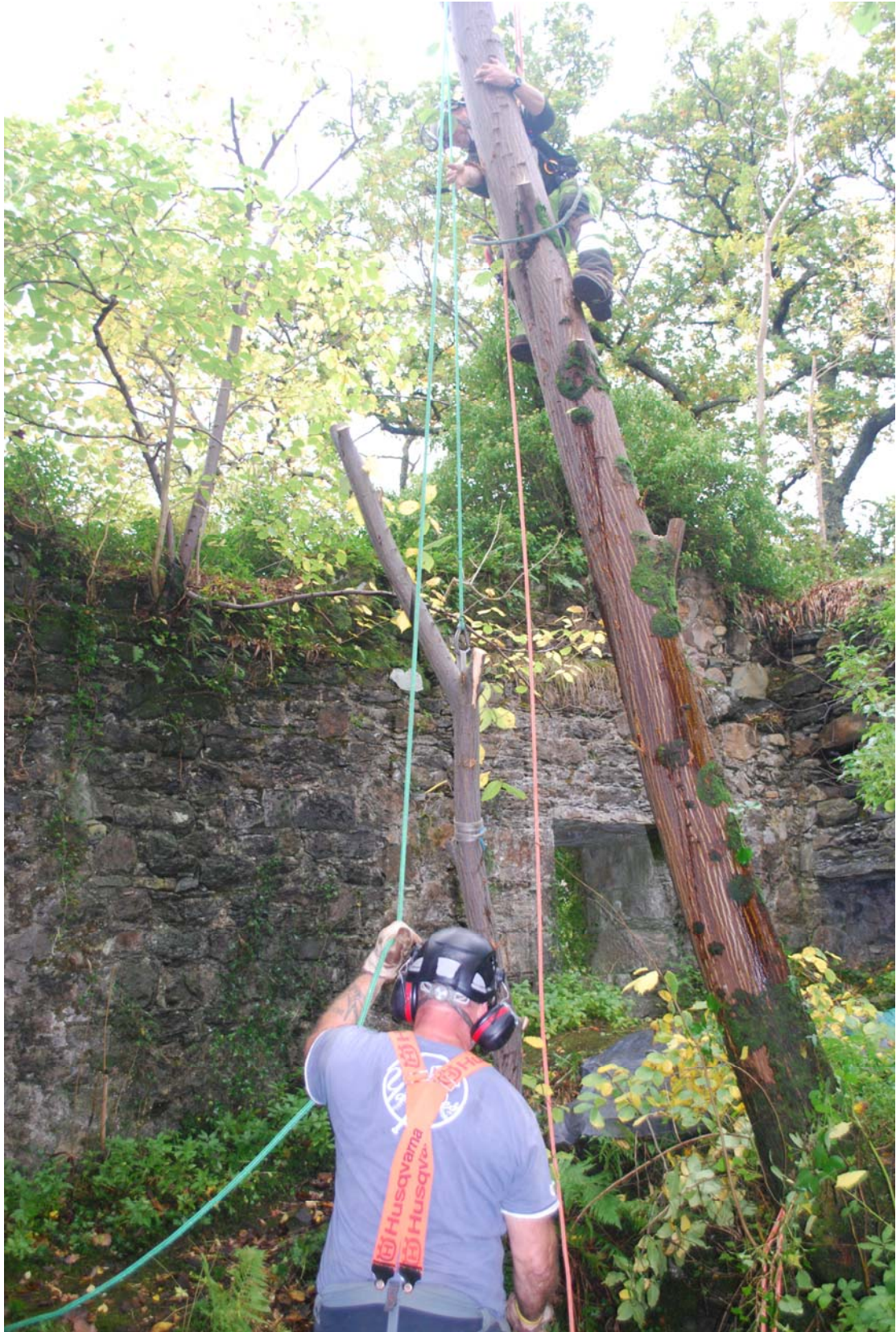
View to the S of Liam MacKenzie (in tree) and Derek Triplett lowering limbs from the Scot's Elm on a pulley system to avoid damage to the structure.
